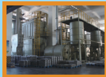
Lead power preparing
